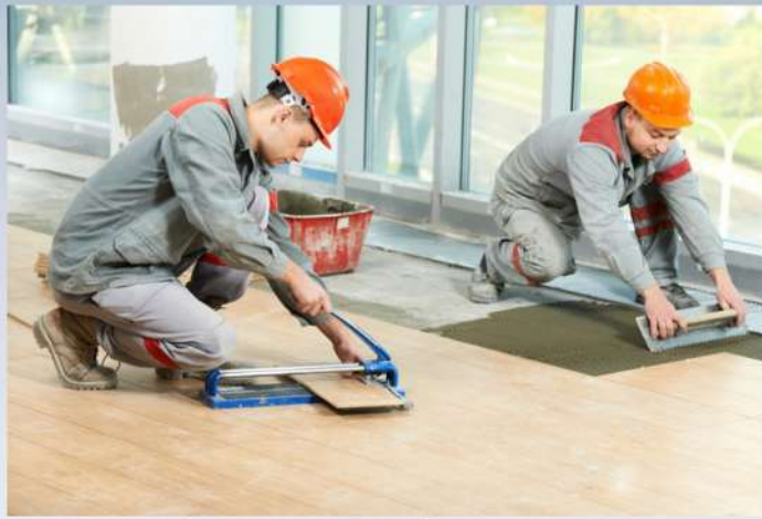
TILES AND GRANITE WORKS
