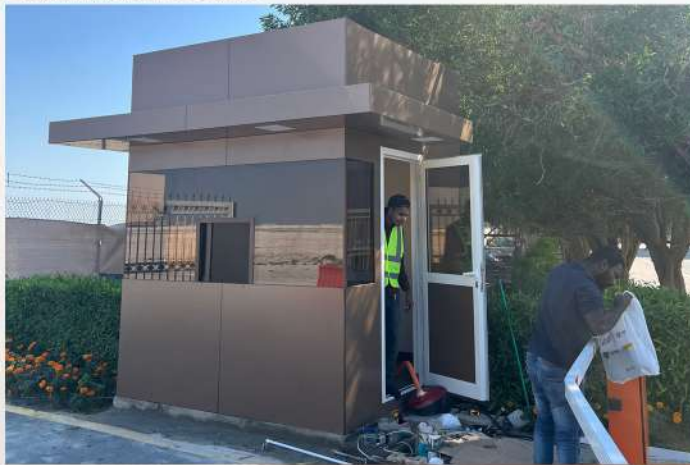
SECURITY GUARD HOUSES FABRICATION
