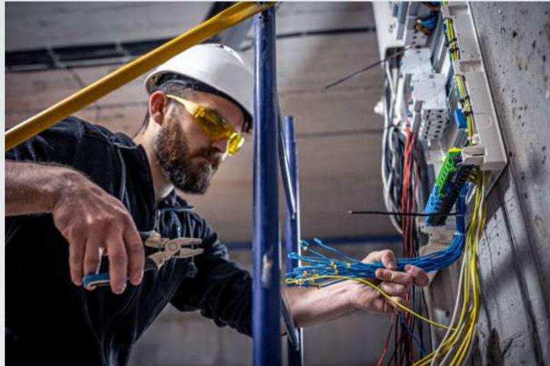
GENERAL ELECTRICAL WORKS
